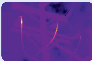
Distribution line faults
