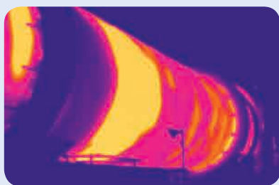
Damaged refractory lining
