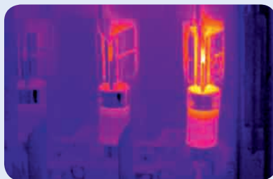
Faulty fuse connection
