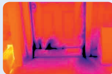
Cold air leaks
